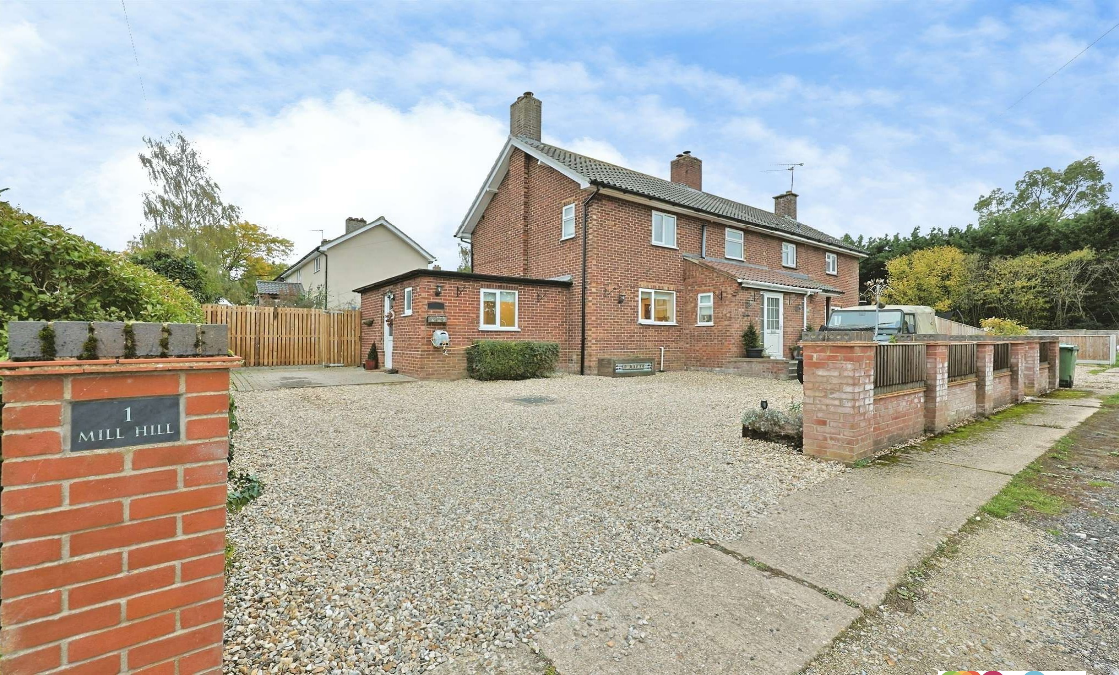
Mill Hill, Bradenham, IP25 7QW
