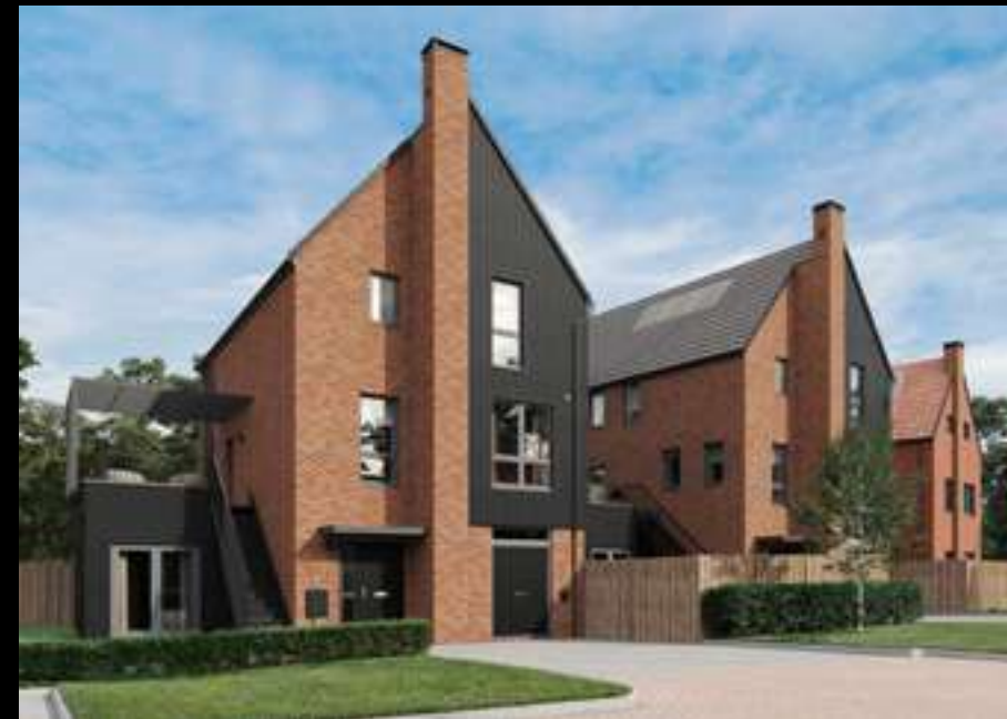
The Railton 4 bedroom detached home
