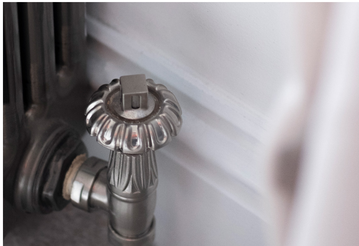
Decorative art deco TRVs and steel column radiators
