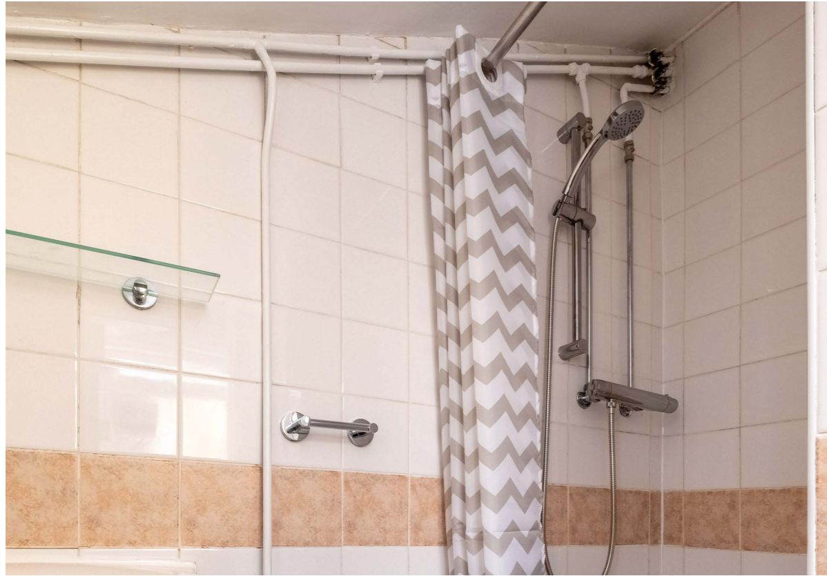
Ground floor shower room detail
