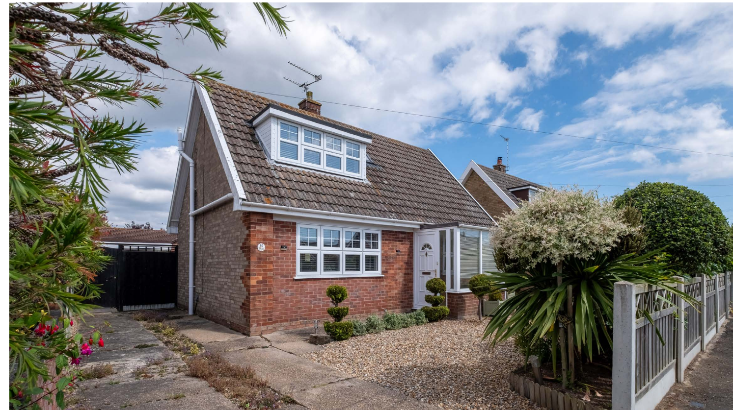
Main facade and driveway
