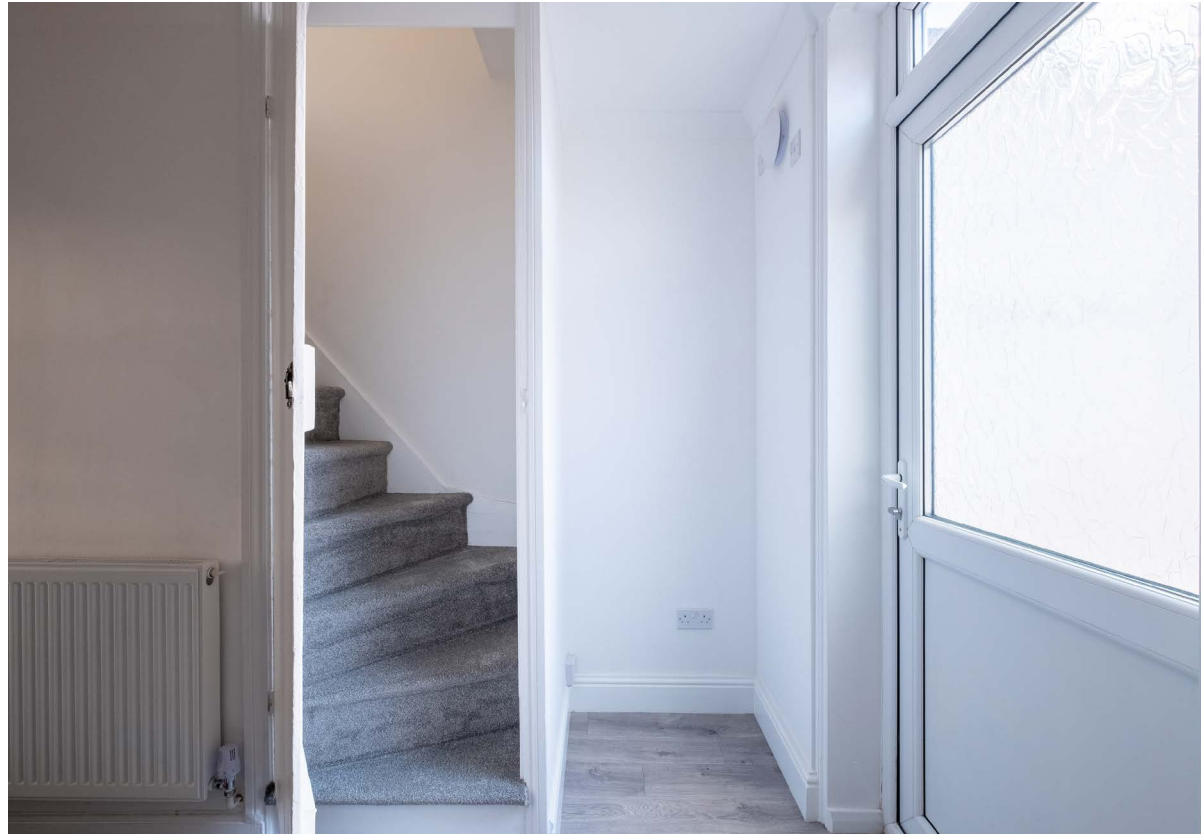
Enclosed staircase leading to first floor.
