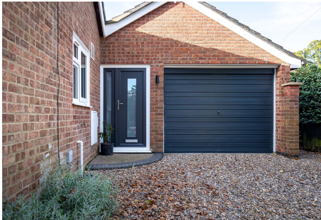
Private gravelled driveway leading to garage
