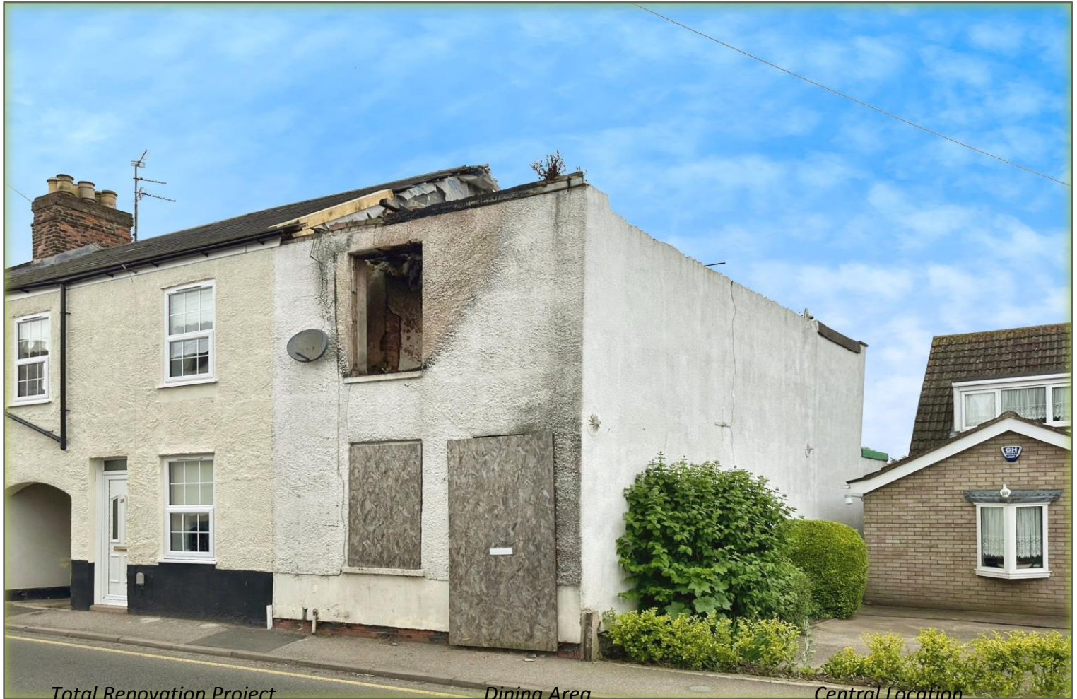
Total Renovation Project
