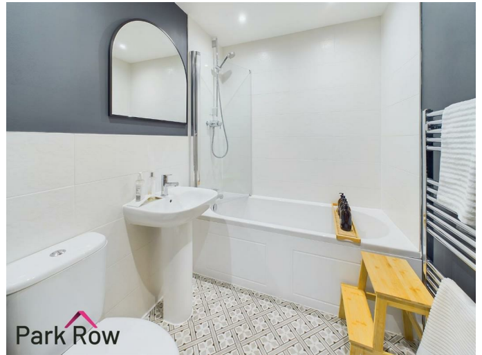
Includes a white suite comprising: panel bath with chrome tap over and mains shower above with glass shower screen, pedestal handbasin with chrome tap over, close coupled w/c, chrome heated towel rail, spotlights to the ceiling and is fully tiled around the bath area and half tiled around the handbasin and w/c.
