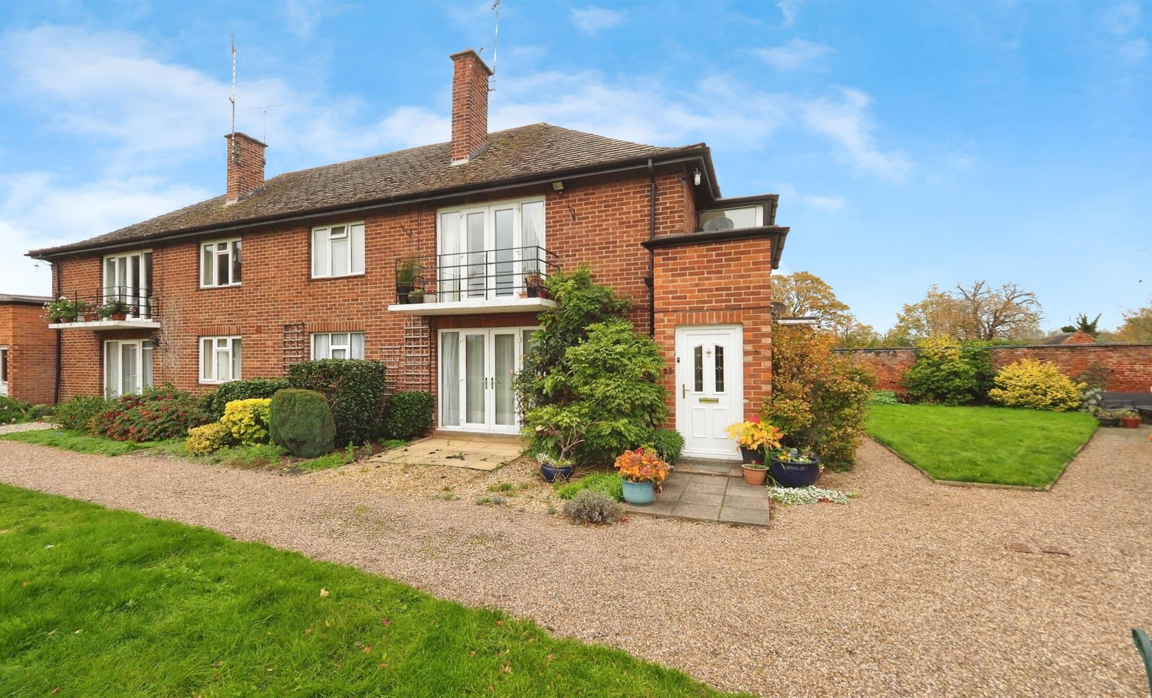
Manor Court Flats Church Lane Barrow-On-Trent Derby
