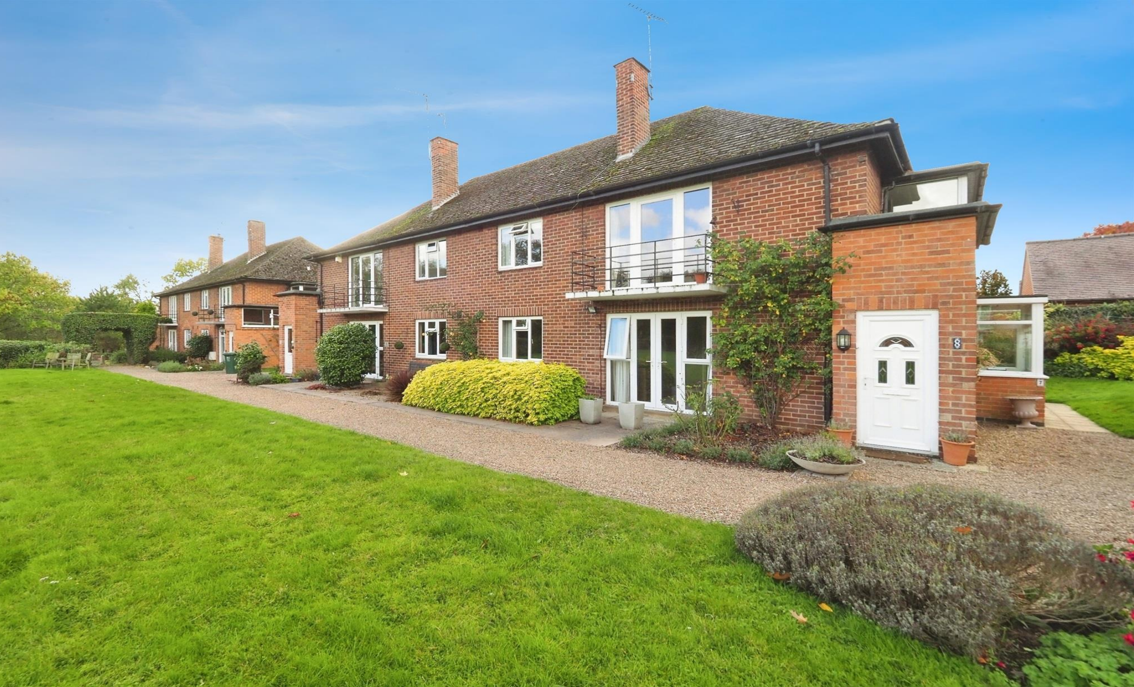
Manor Court Flats Church Lane Barrow-On-Trent Derby
