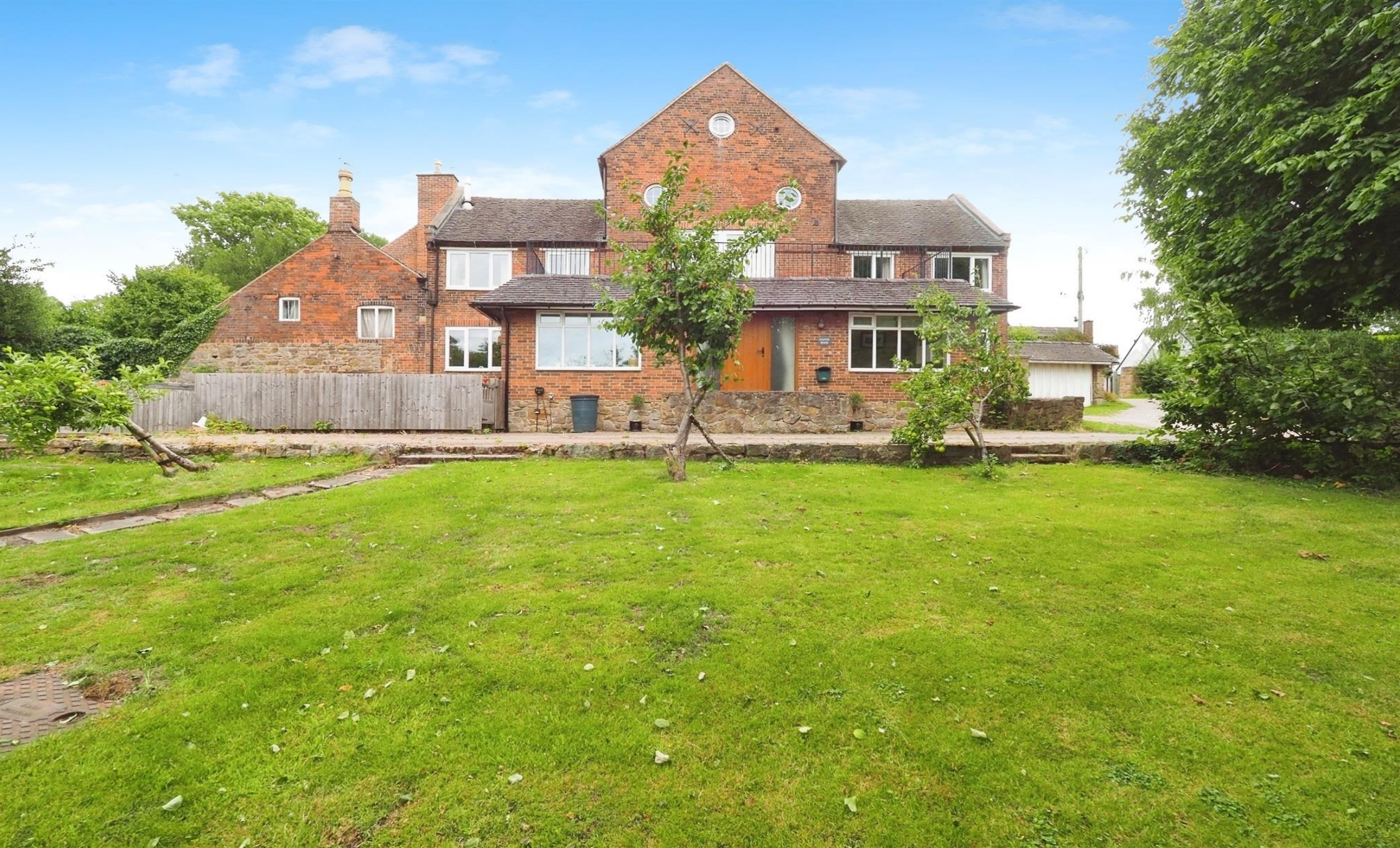
Stanton House Ingleby Road Stanton-By-Bridge Derby
