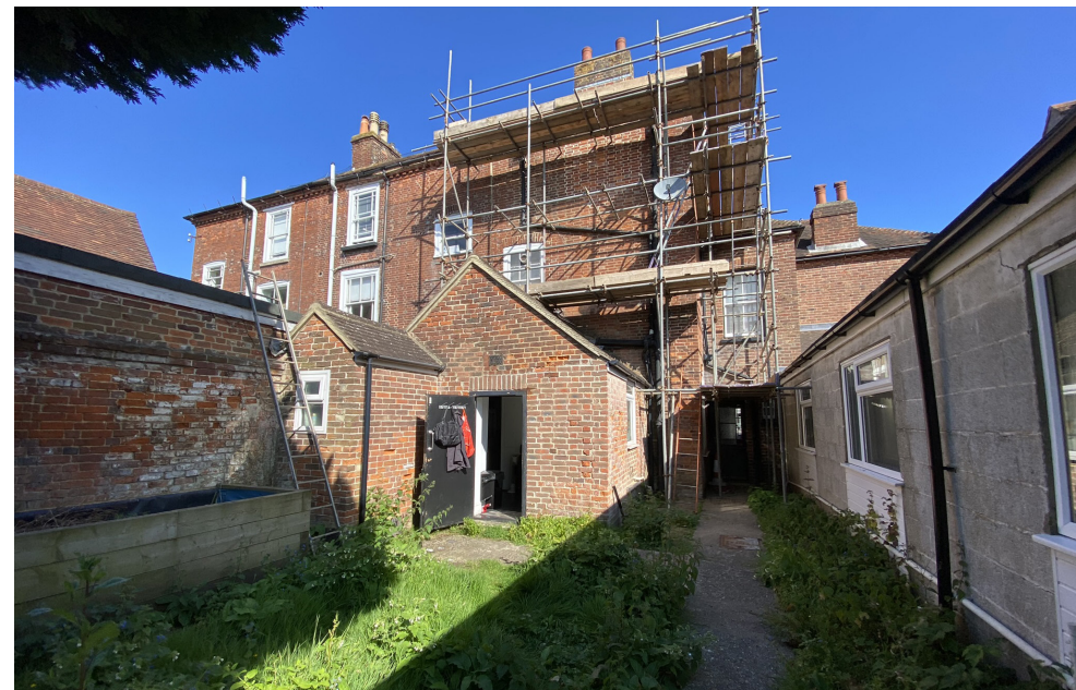
Works completed but scaffolding still in place due to nesting gulls.
