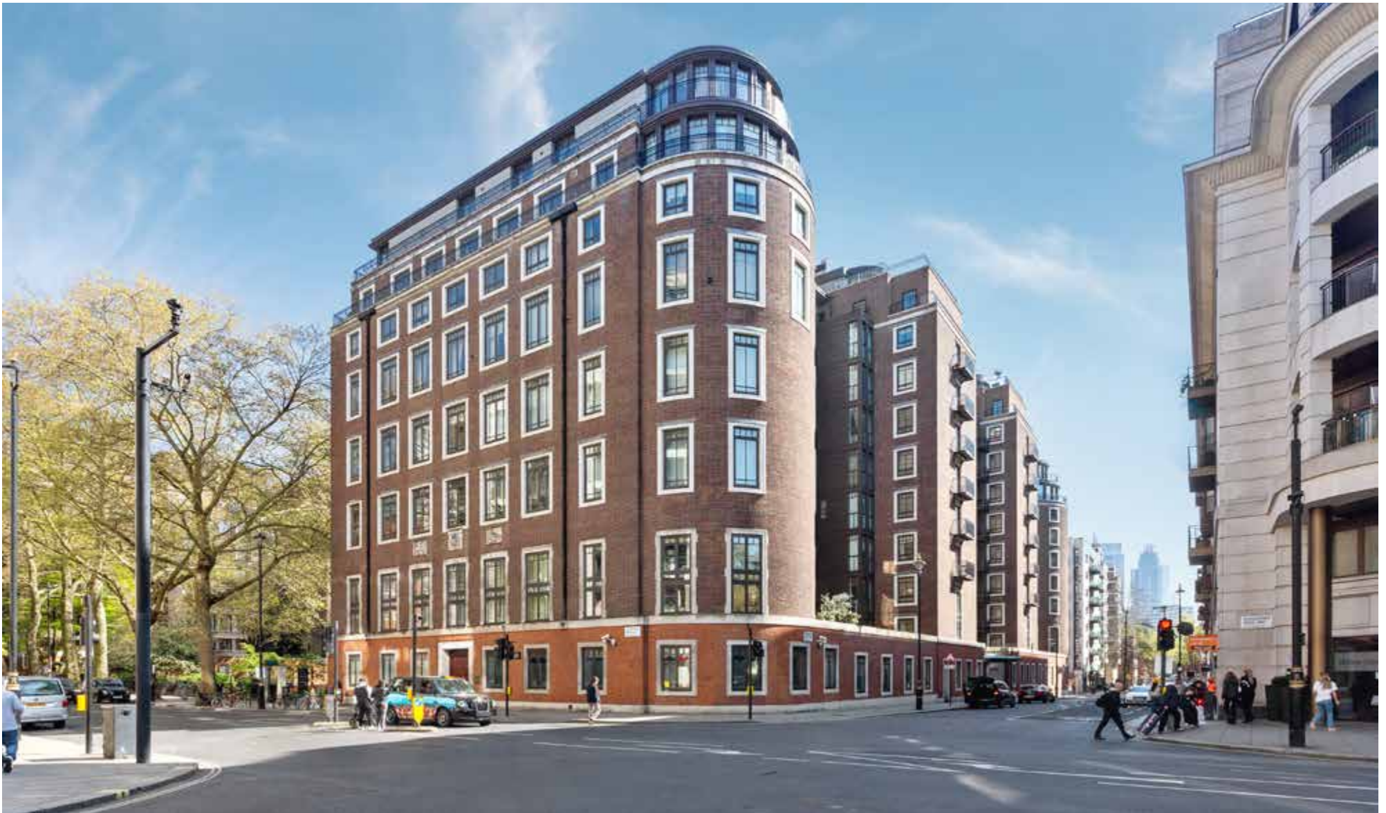
St Johns Building Marsham Street SW1P
