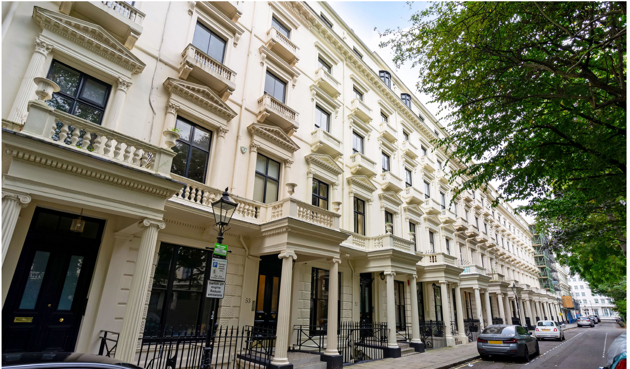
Queens Gardens Bayswater W2
