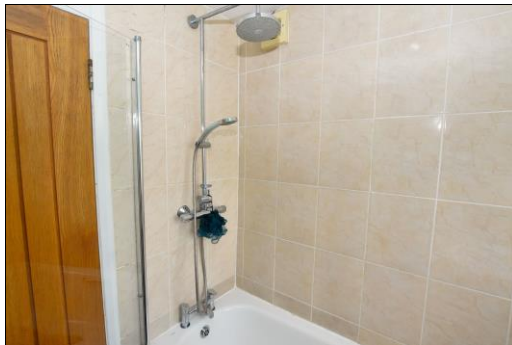
Bathroom shower detail
