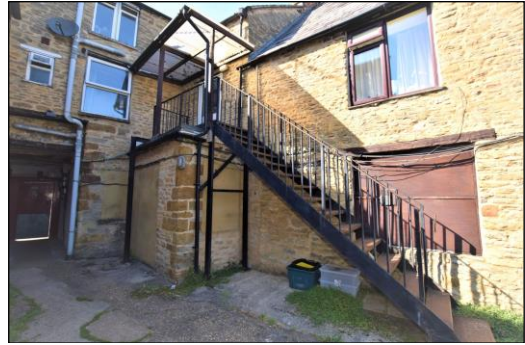
External staircase in Mews
