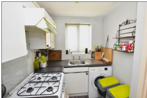
Old Kitchen ( Being Replaced)
