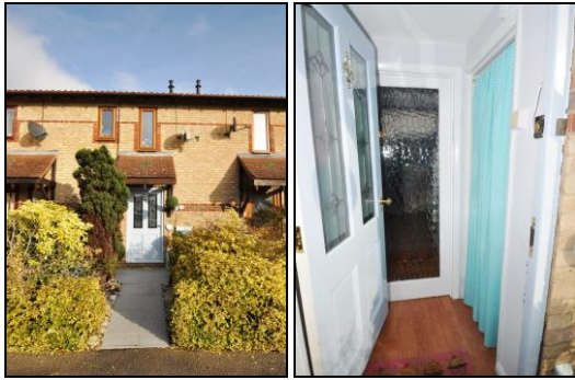
Front Elevation & Entrance Lobby
