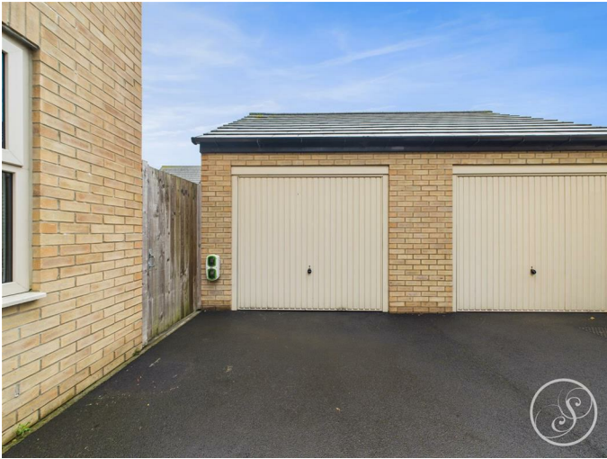
Power and lights.
