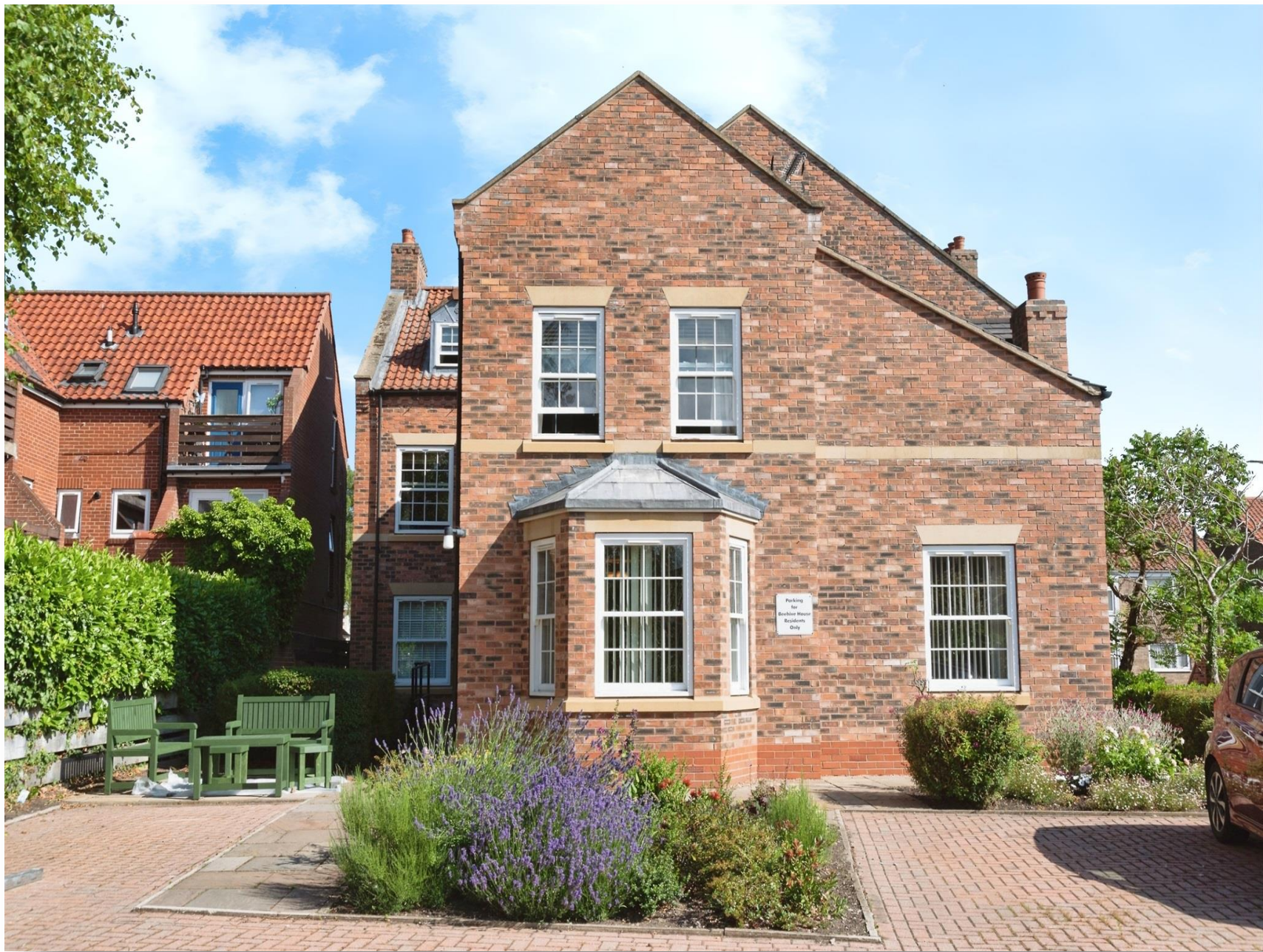
Beehive House, Keldgate Bar, Beverley, HU17 8AG
