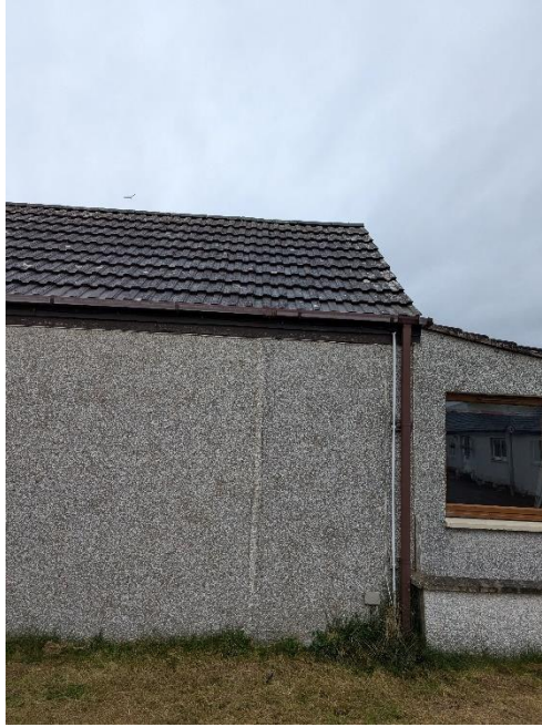
Photograph 7 – Cracking to elevation adjacent to neighbouring property
