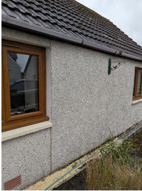
Photograph 3 – Joint in render at front elevation
