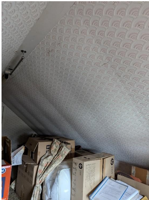
Photograph 12 – Sagging between rafters in loft
