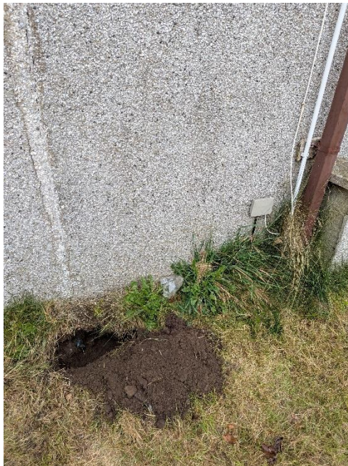
Photograph 8 – Hand dig at foundation
