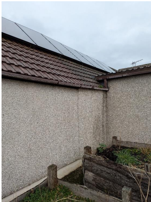
Photograph 4 – Joint in render at rear elevation
