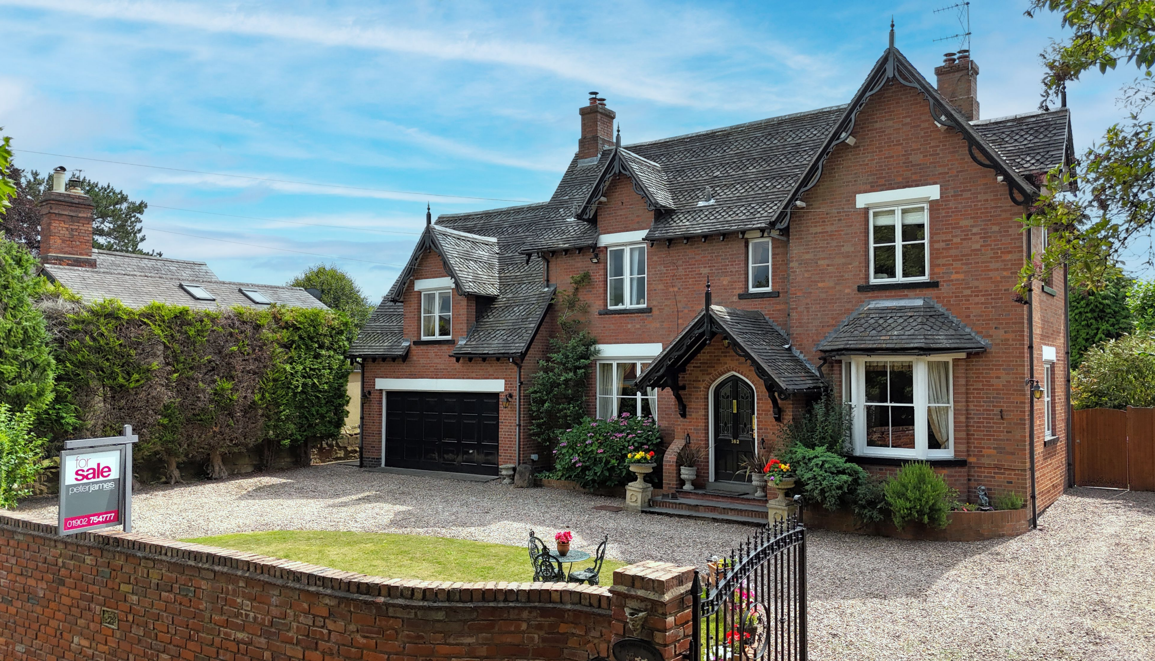
The Coach House, 162 Wergs Road Tettenhall, WV6 7LB
