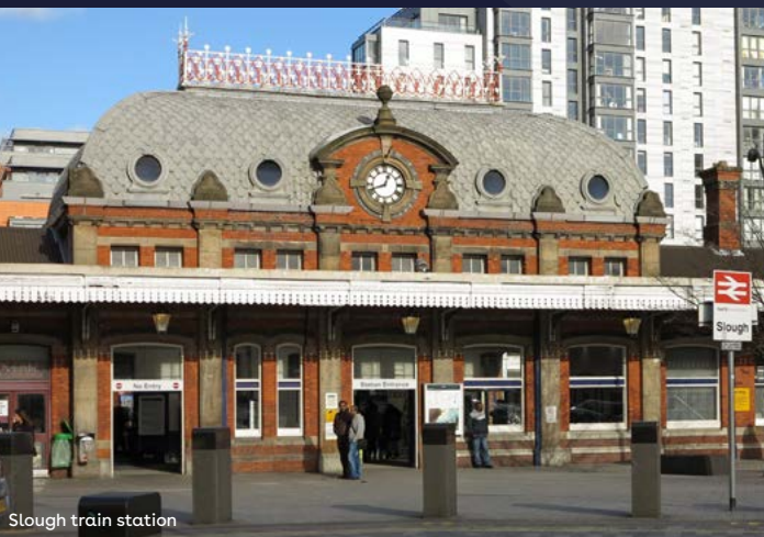
Slough train station
