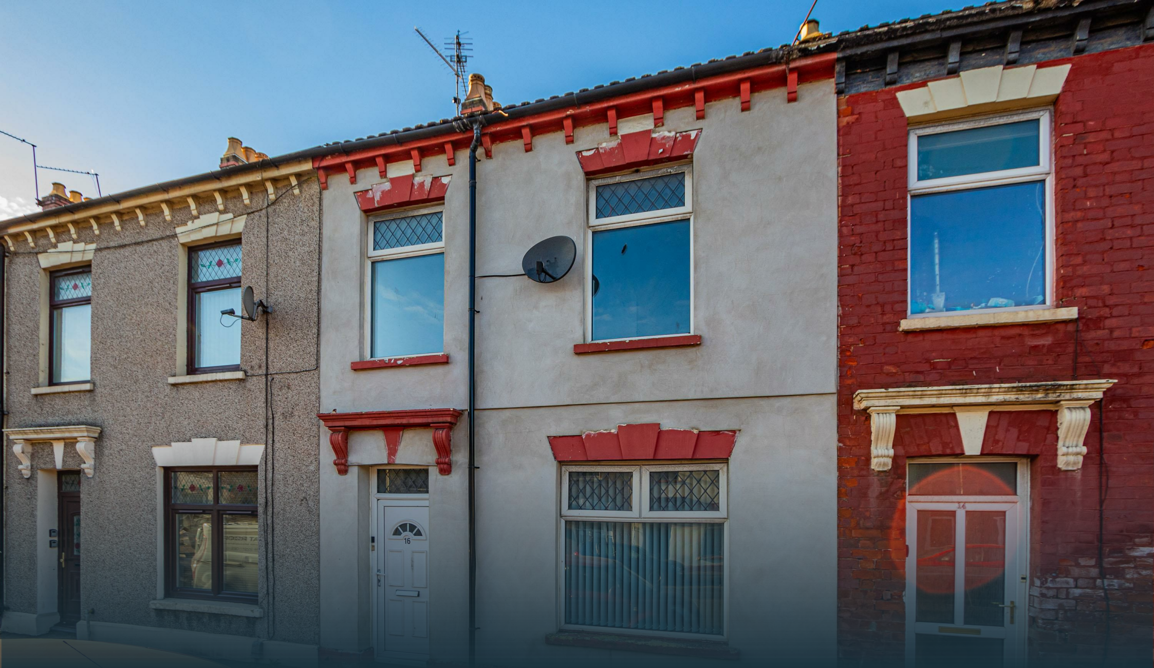
LOWER CATHEDRAL ROAD RIVERSIDE
