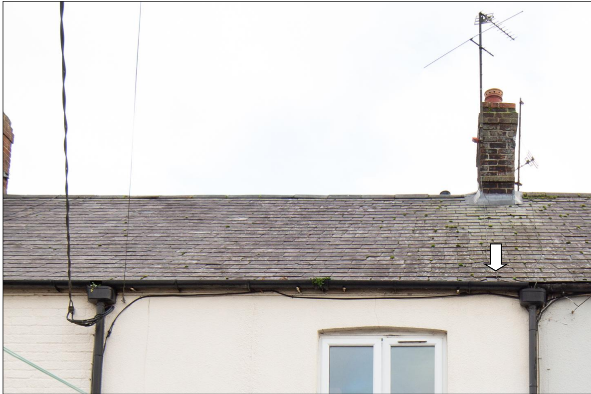
Roof close-up, slipped tile indicated by arrow
