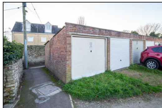
Garage in Block
