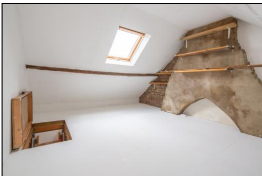
Lined & Floored Loft Space
