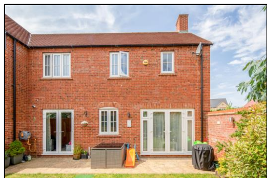
Rear Elevation and Patio
