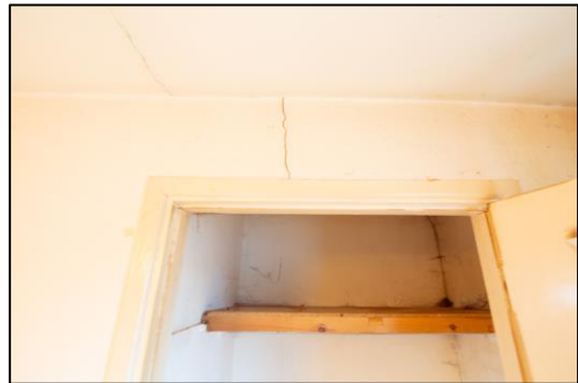
Settlement Cracking
