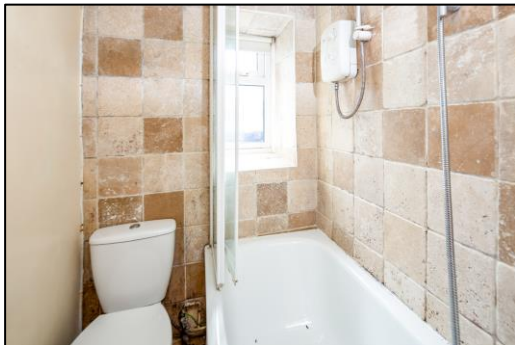
Ground Floor Bathroom
