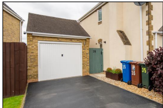
Garage and Driveway
