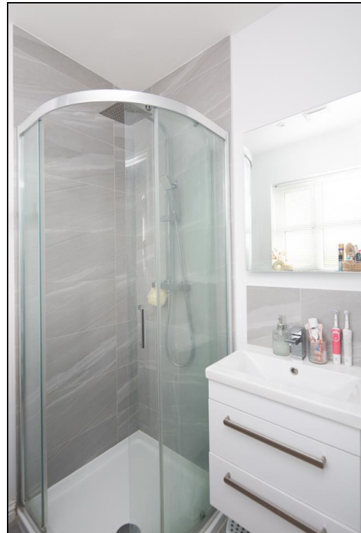
Re-fitted En-Suite Shower
