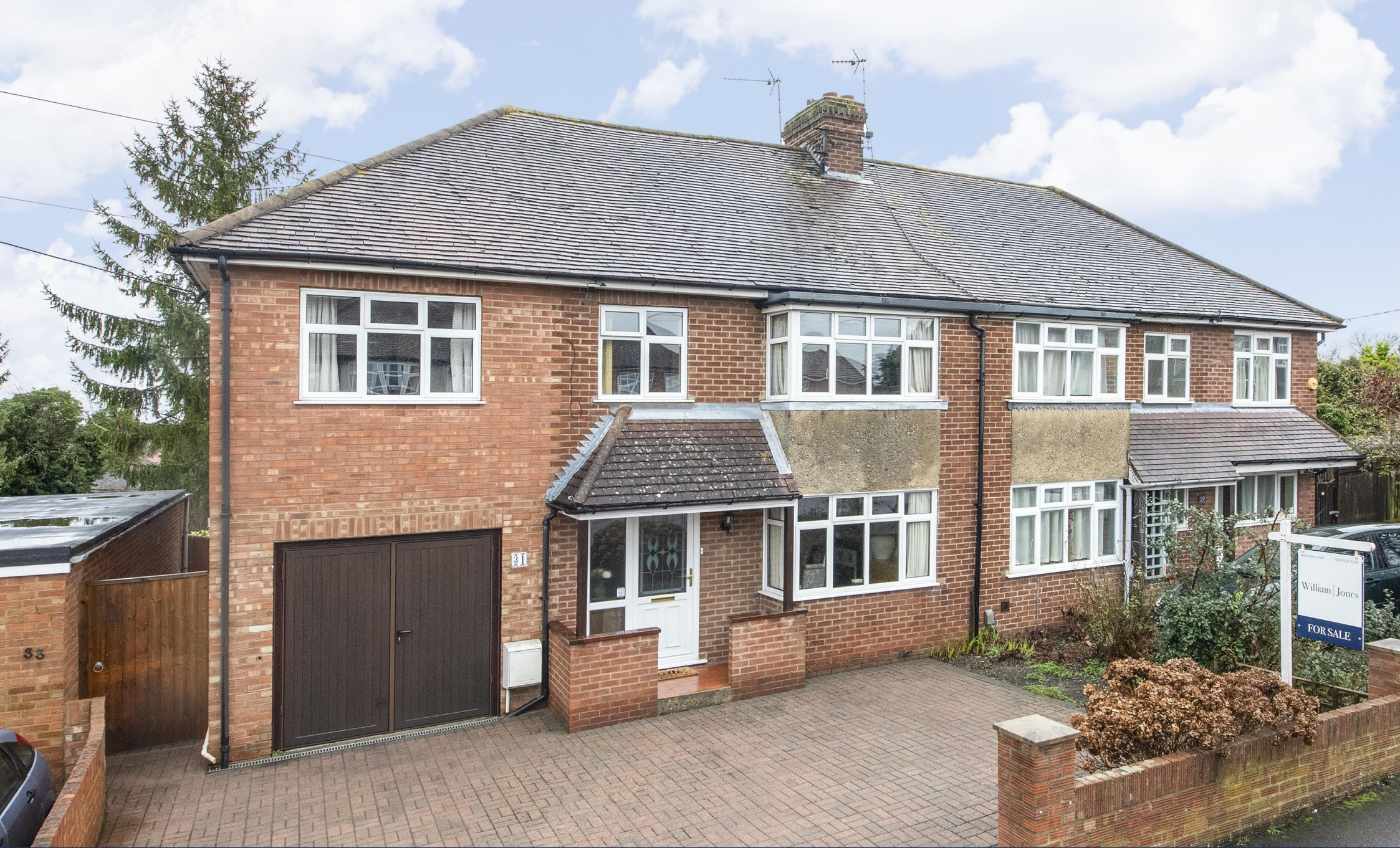
31 Haydon Road, Didcot, Oxfordshire, OX11 7JA
