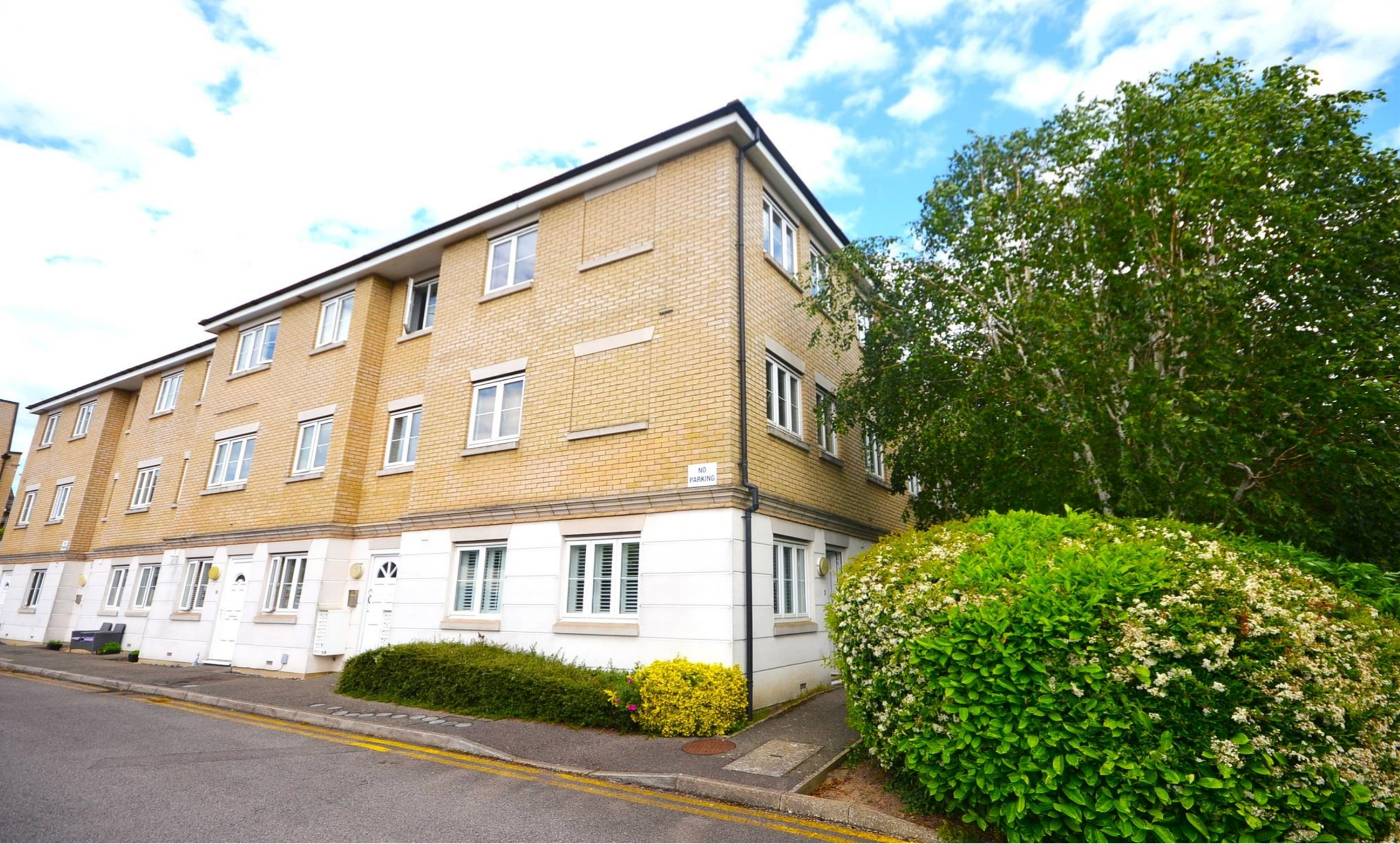
Timber Yard, Station Approach, Braintree, CM7 3TB
