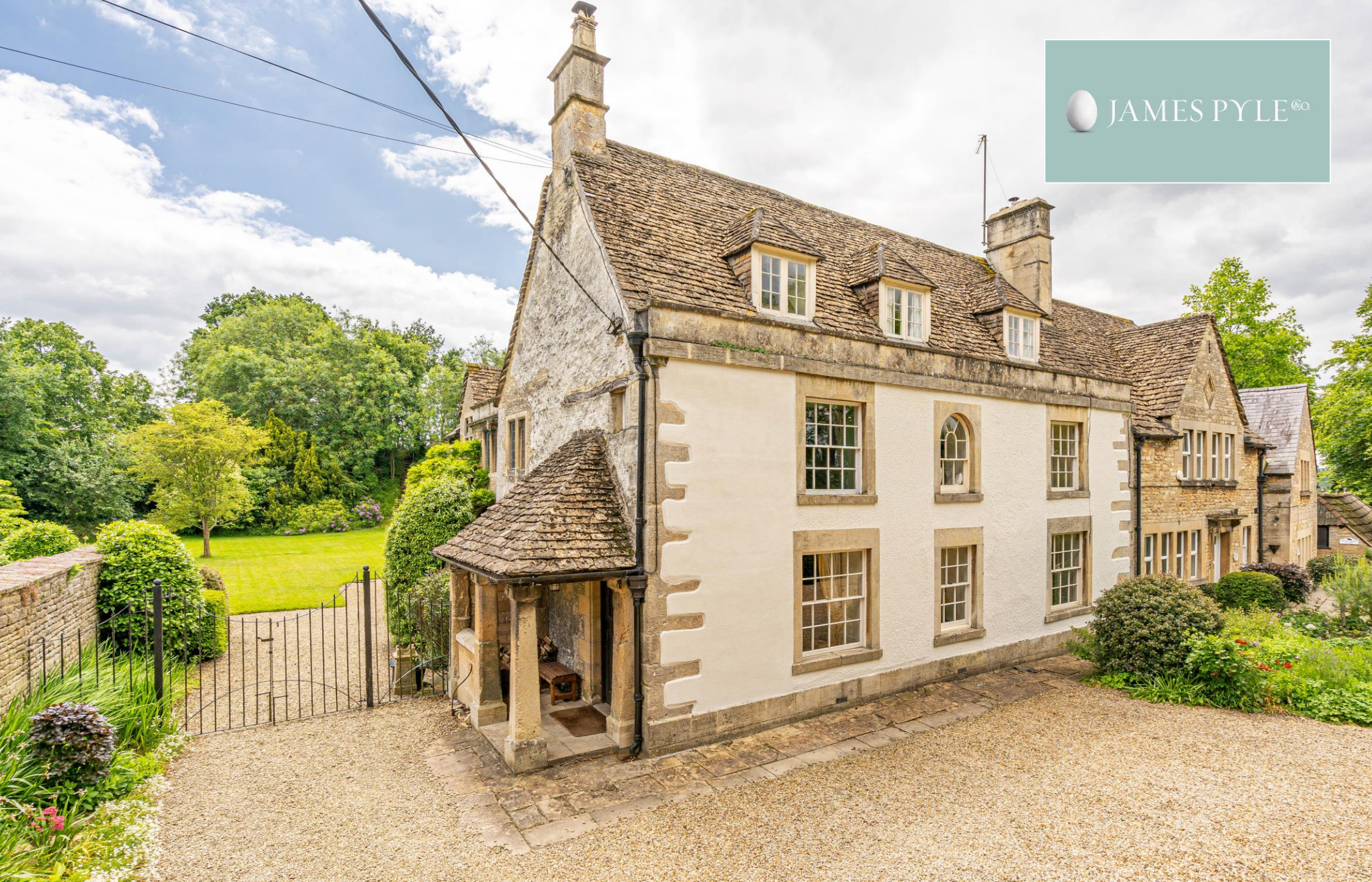
Lowden Manor House, Lowden Hill, Chippenham, Wiltshire, SN15 2BX
