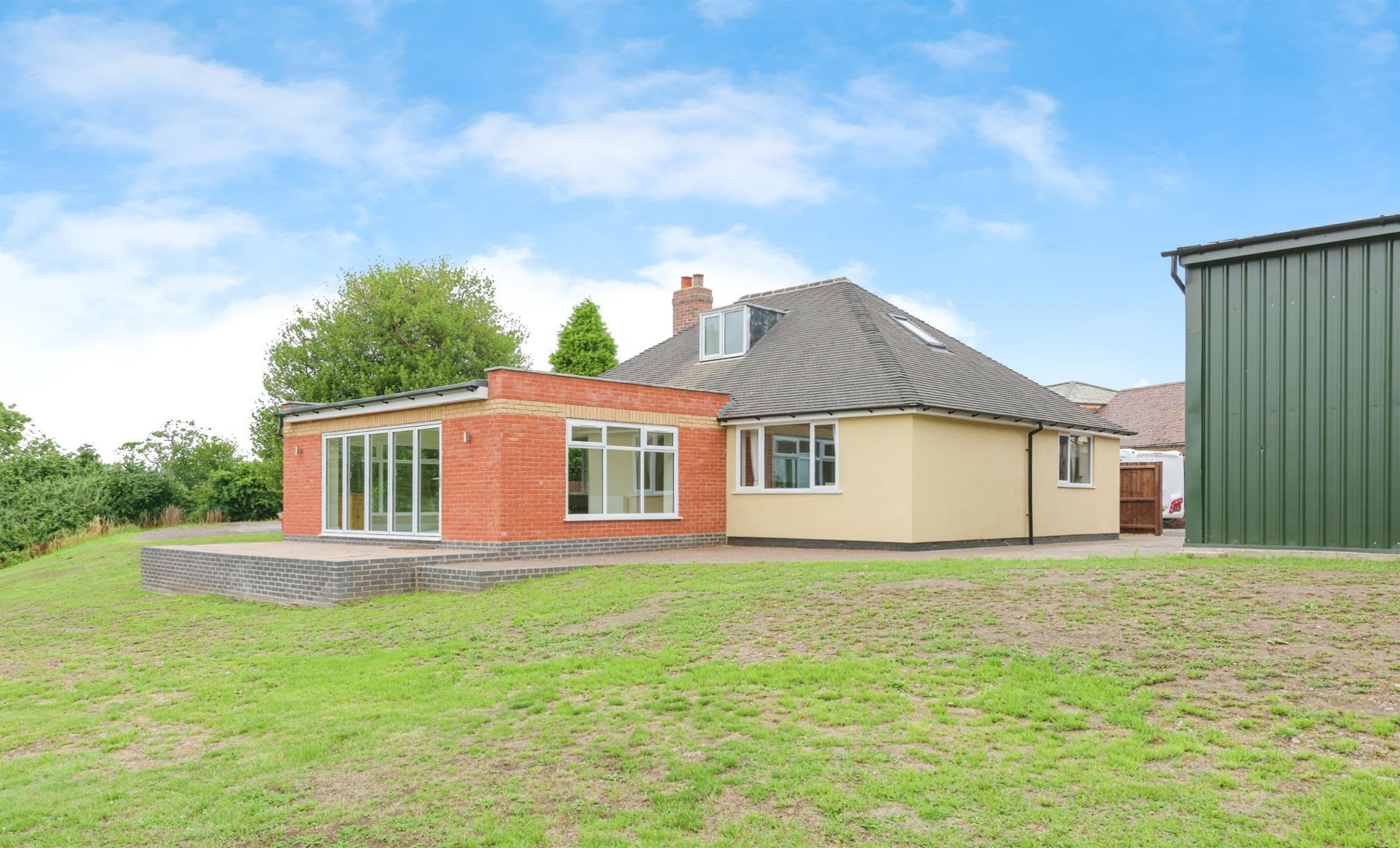
Tame View, Cliff Hall Lane, Cliff, Tamworth
