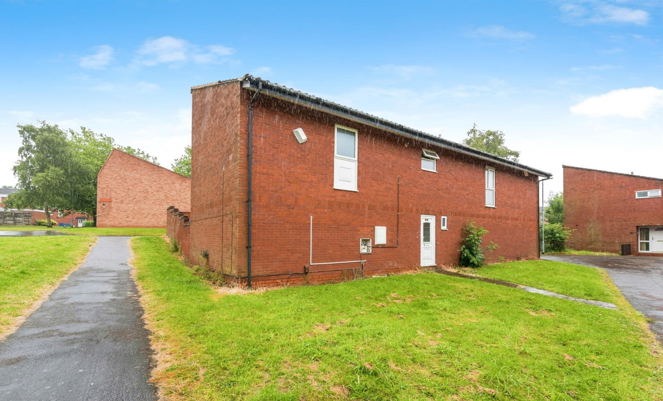
Camhouses, Wilnecote Tamworth
