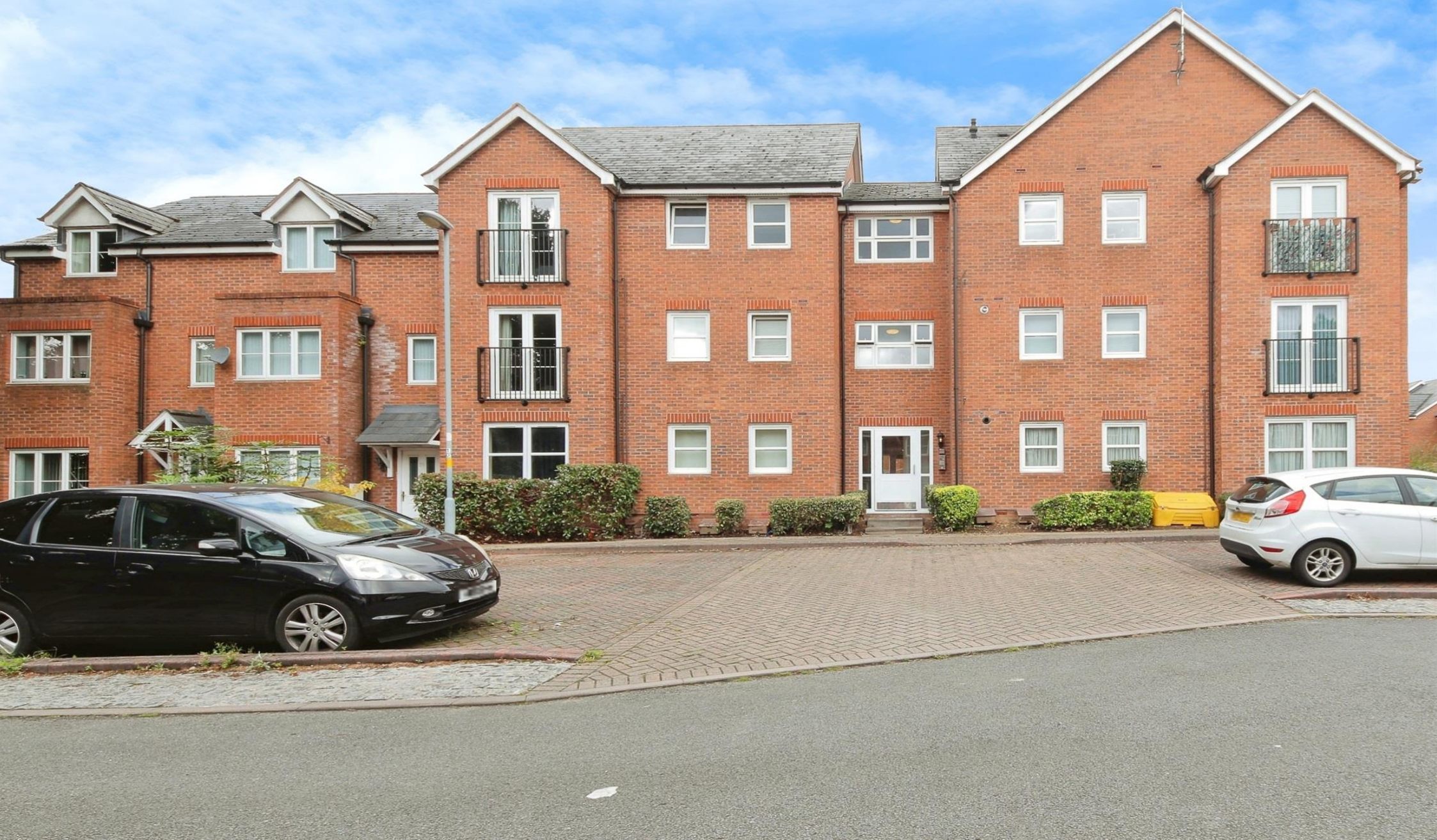
Canal Court, Birmingham
