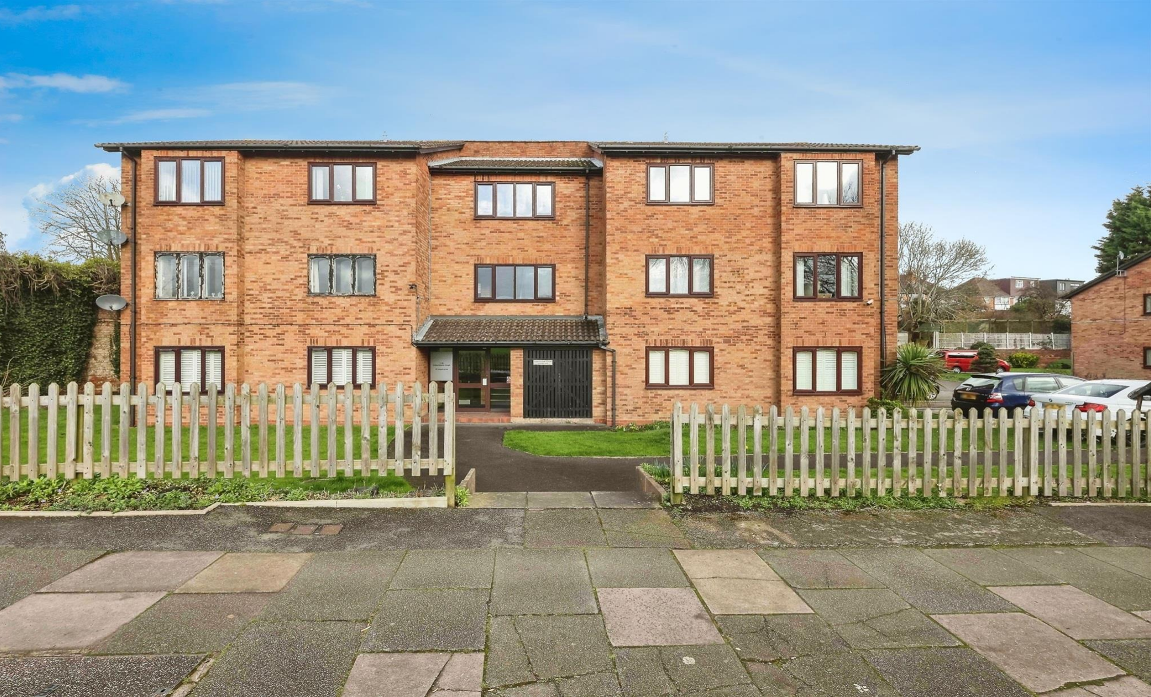
Gilberstone Court Moat Lane, Yardley Birmingham
