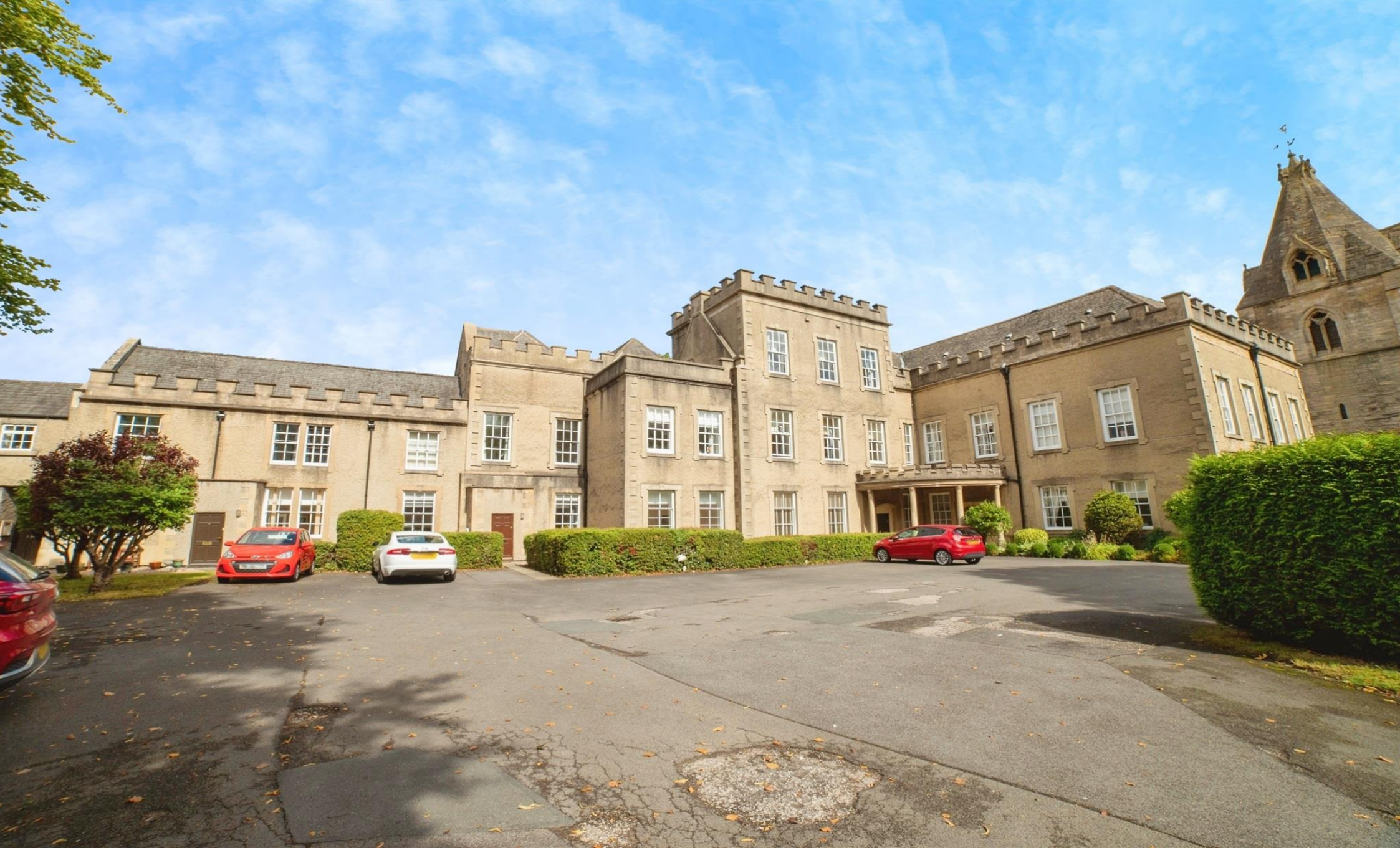
Manor House Mansfield Woodhouse Mansfield
