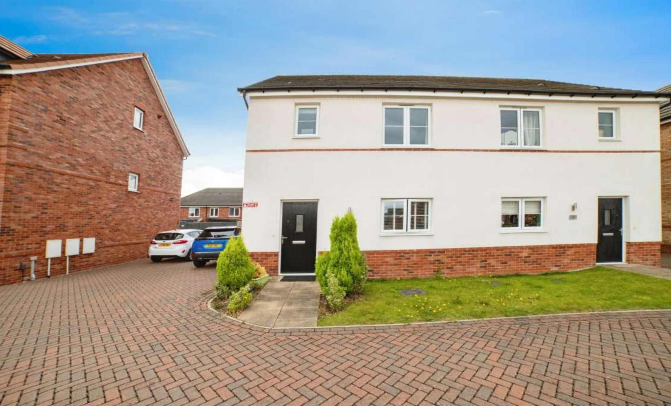
Rosebay Gardens Clipstone Village Mansfield
