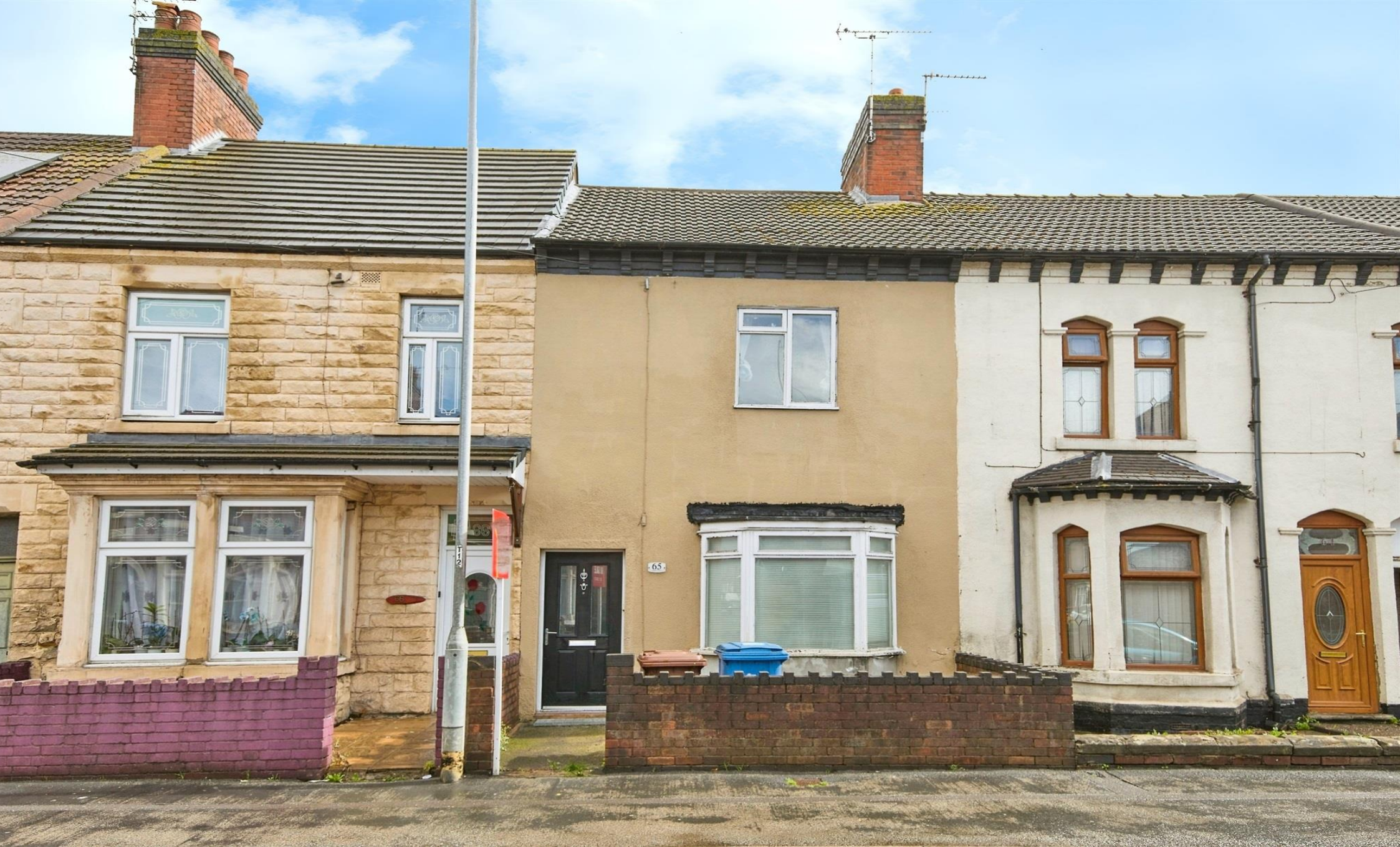
Shobnall Street, Burton-On-Trent
