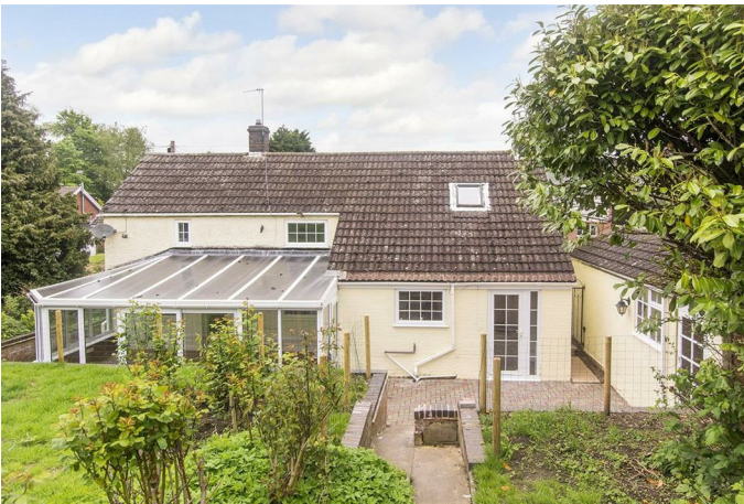
Rear of House
