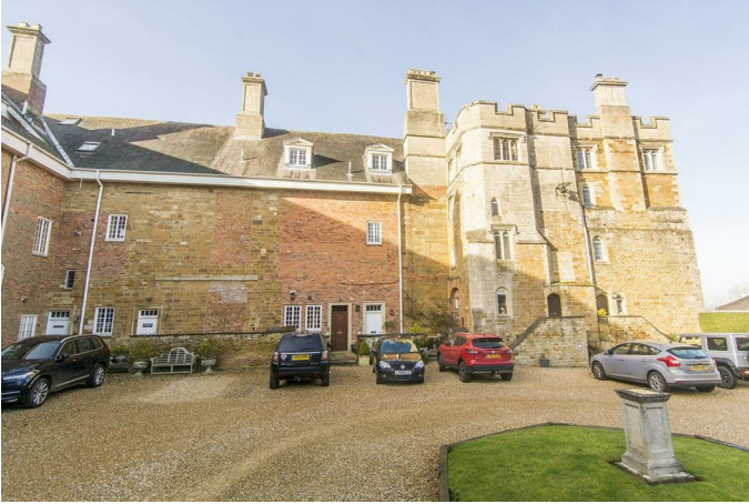
Communal Parking Area
