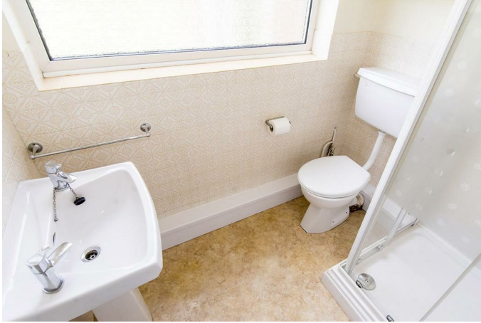
Downstairs Shower Room 6'5 x 4'10 (1.96m x 1.47m)
