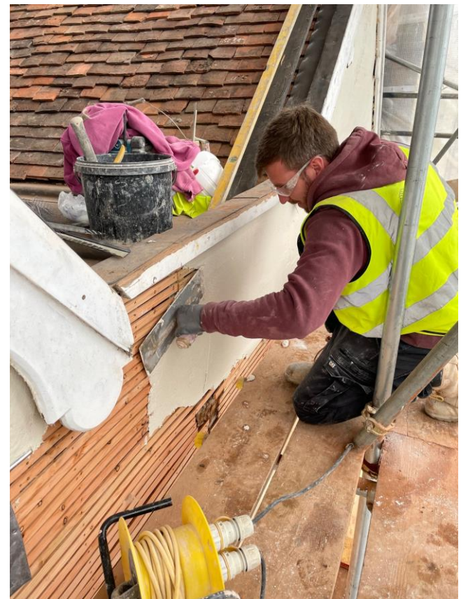
Tommy Scott, of Gower Brothers, lime plastering on softwood laths externally.
