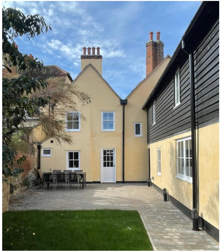
Right: The rear elevation following renovation, including the removal of a modern conservatory, replacement windows, re-rendering, and landscaping
