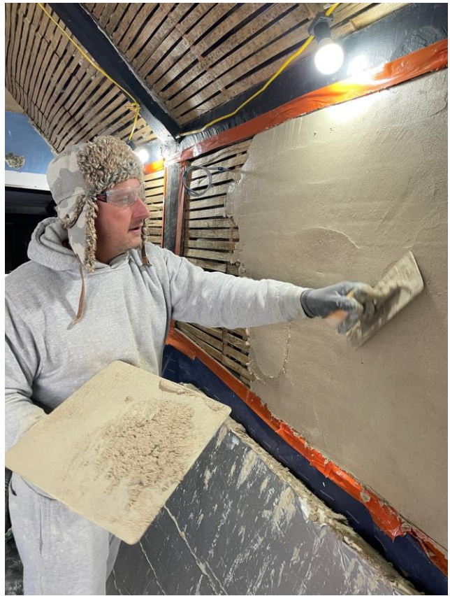
Jason Root, of Gower Brothers, lime plastering on oak laths in the hall chamber.
