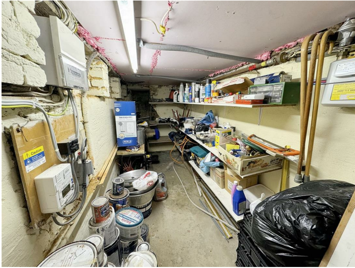
wall mounted gas meter, electric meter and consumer unit.
