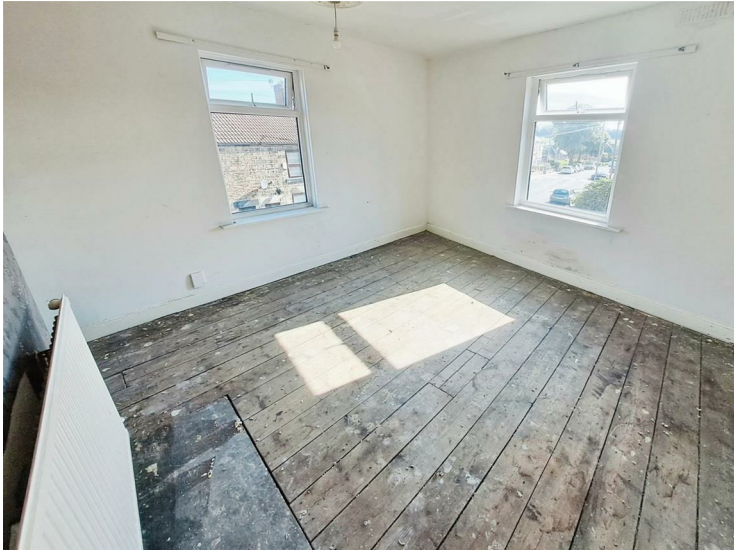
Having a window and a radiator.
