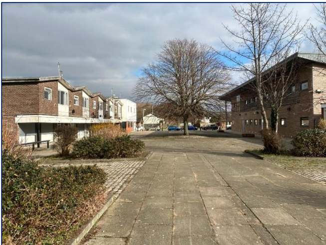
WEST APPROACH SANDBROOK WAY
