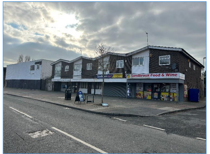
NORTH APPROACH FROM SANDBROOK RD
