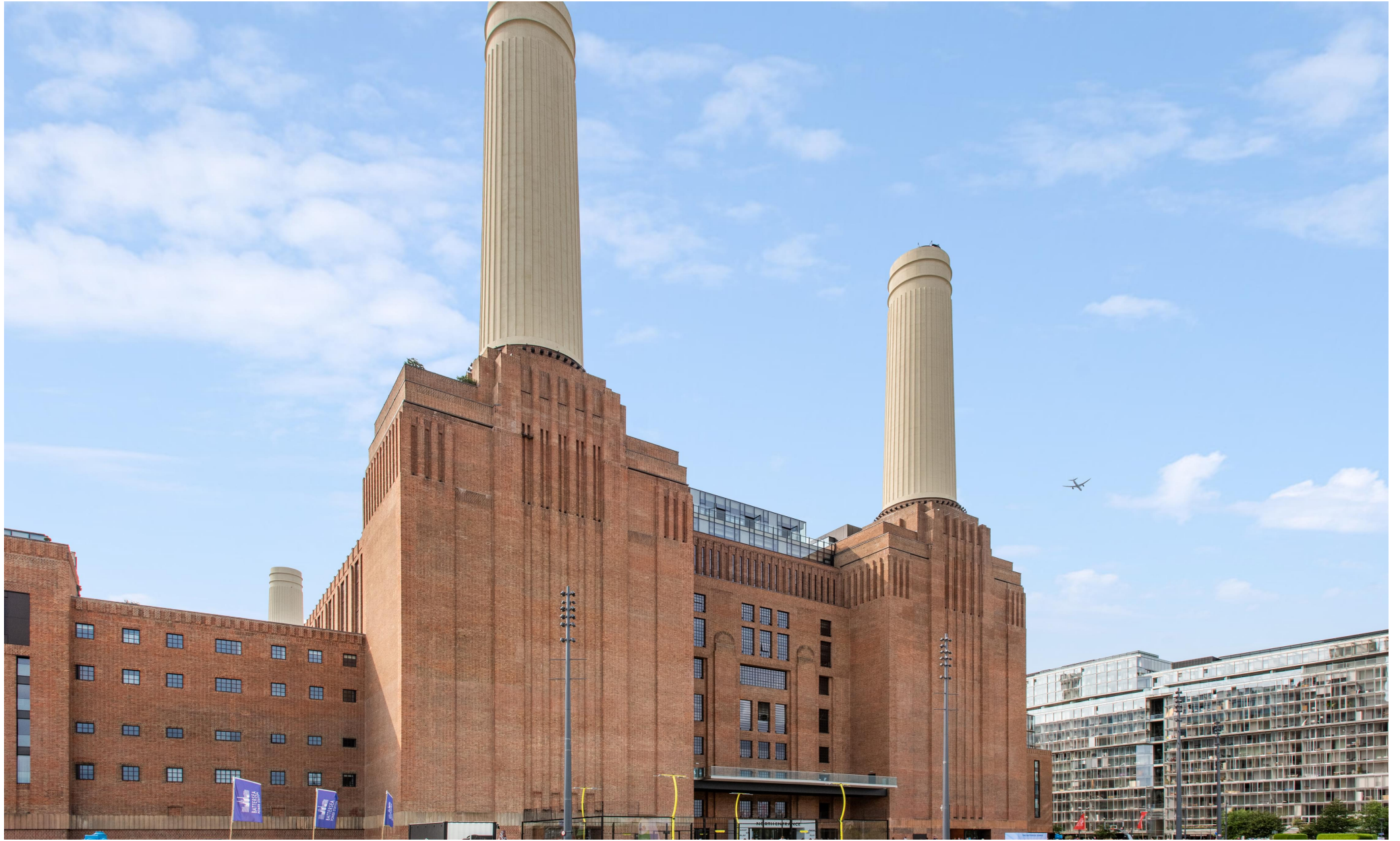
Switch House East, Battersea Power Station SW11
